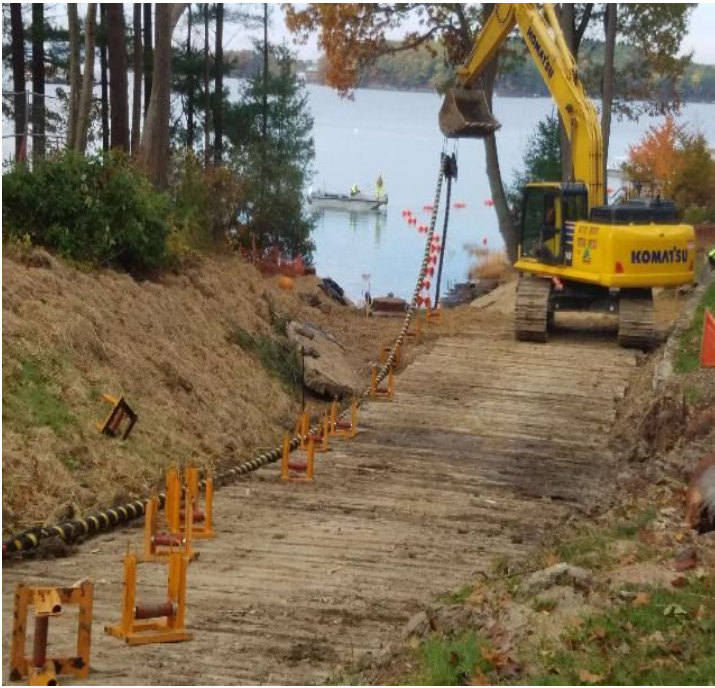
Fig 9: Pulling the cable at the Getchell property. Viewing east. (10-22-19).
