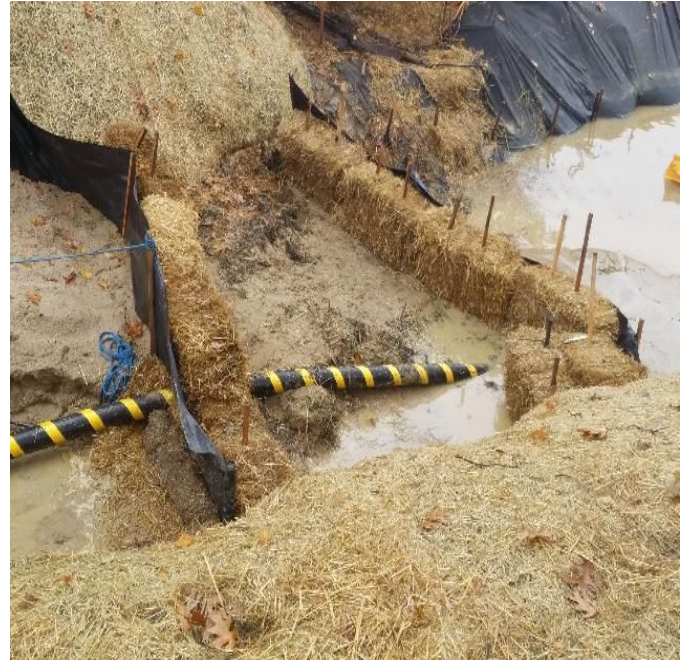
Fig 22: Temporary repairs made to sediment and erosion controls at Beswick property. (10-23-19).
