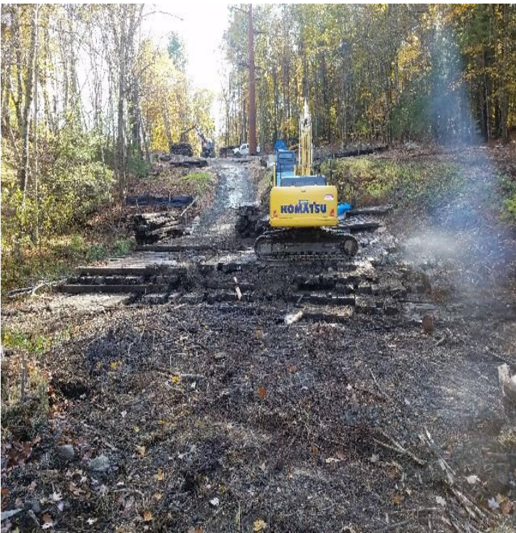
Fig 23: JCR removing timber mats around Str. 28. Viewing south. (10-23-19).
