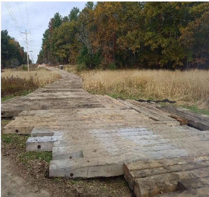
Fig 11: Matted access road through wetland DW6. Viewing west. (10-22-19).
