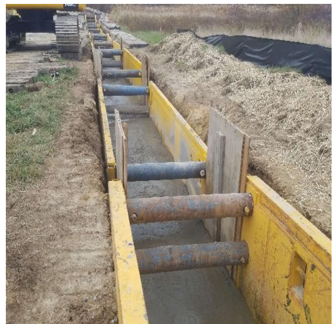
Fig 12: Poured duct bank in trench at Frink farm. Viewing east. (10-22-19).
