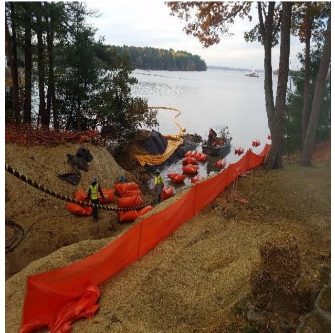
Fig 10: Pulling the cable at the Getchell property. Viewing east. (10-22-19).
