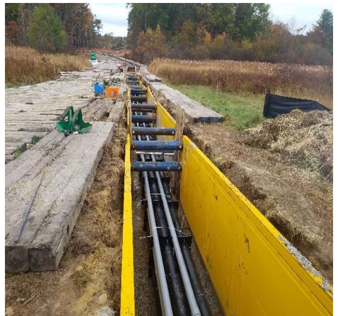
Fig 8: Assembling pipe in trench at Frink farm. Viewing east. (10-22-19).
