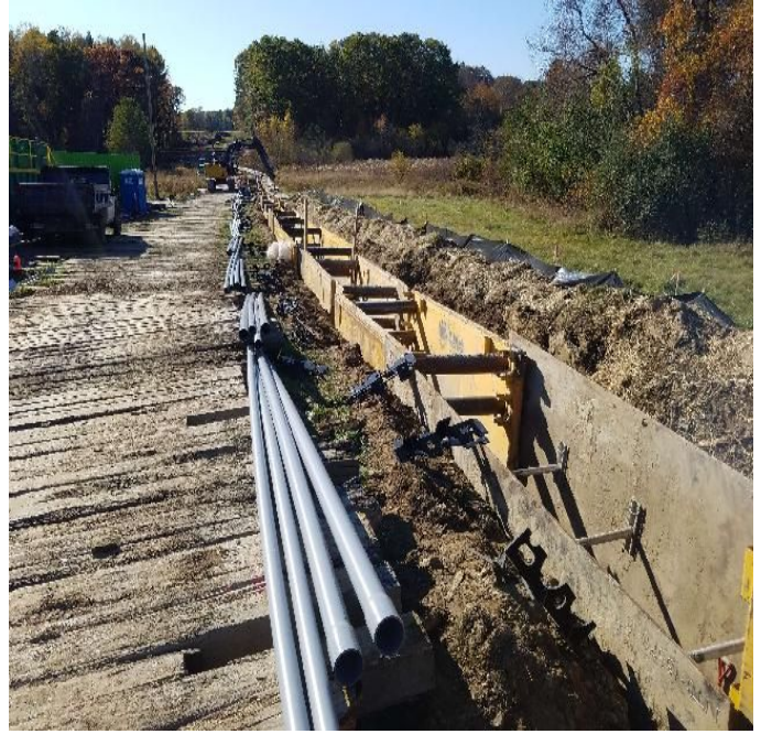
Fig 2: Trenching activities at Frink farm. Viewing east. (10-21-19).
